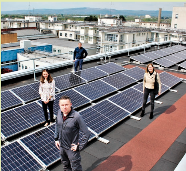
Pictured at the bank of solar PV cells on the roof of the 60-bed block at UHL; Kevin Mahoney, Rachel Keating, Clodagh Hanratty and Niall Joyce
