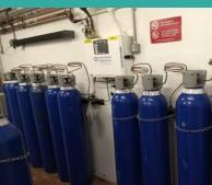
In University Hospital Galway, fixing N<sub>2</sub>O piping leaks led to an 80% reduction in CO<sub>2</sub>e.
