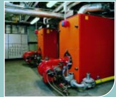
📷 The Boiler House
