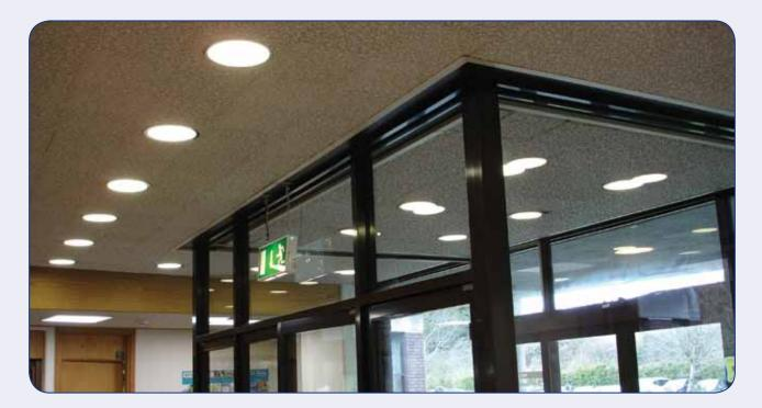
The solution here was to replace a total of 445 sets of 4x18W T8 fittings with 3x14W T5 fittings. The higher efficiency of the T5 lamps/electronic ballasts combined with a higher light output through the new diffusers has allowed a saving of 50% in circuit watts to be achieved per fitting with an improvement in lighting levels in corridor areas.
