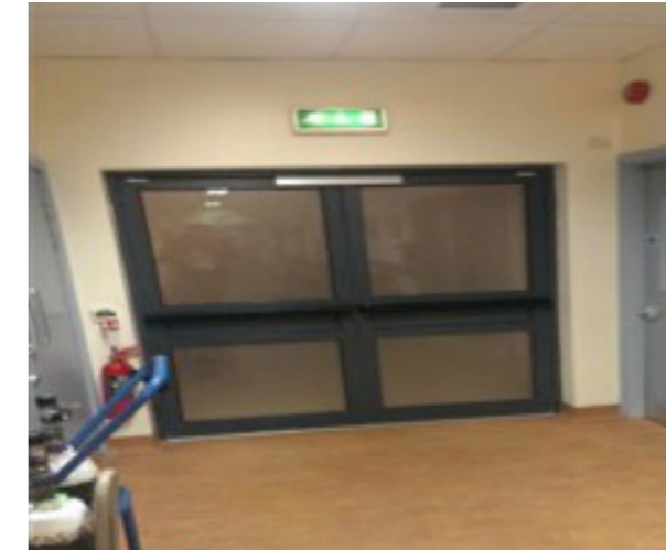
Picture above: Door on ward that concealment will be introduced, however awaiting authorisation from Fire Officer to complete this.
