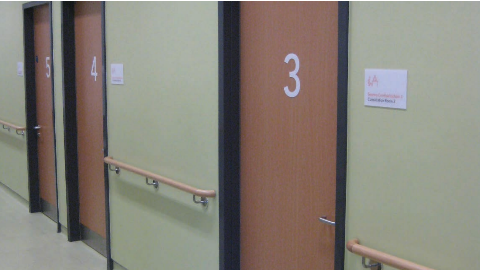
07 Doors, doorframes, and door handles, MISA Building, St. James's Hospital Dublin, Ireland.
