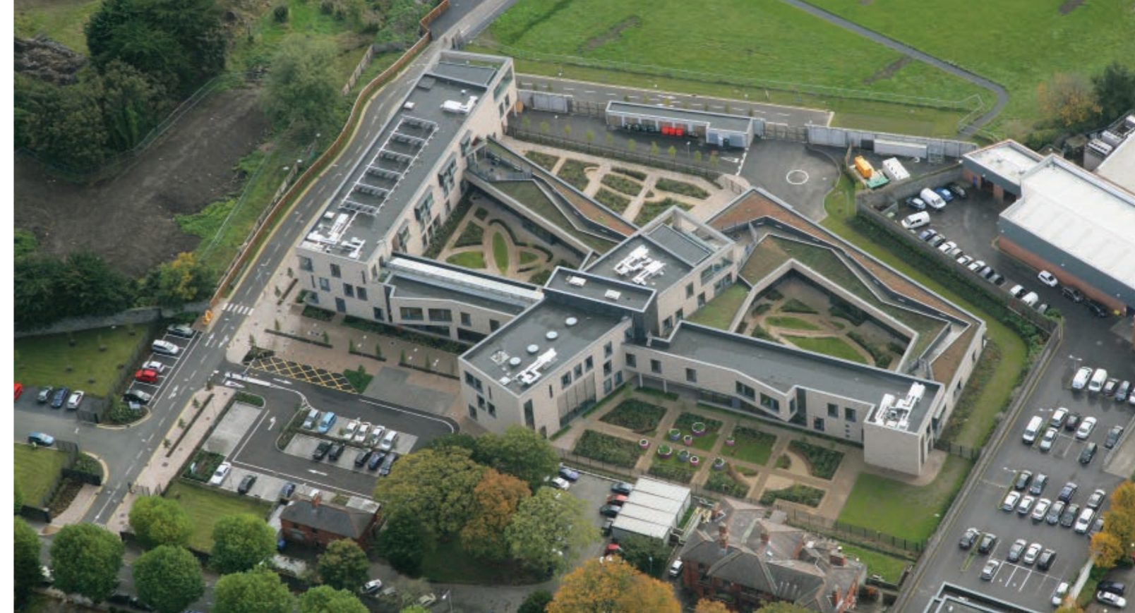
06 Aerial view of Phoenix Care Centre, Granegorman, Dublin 7, Ireland.
