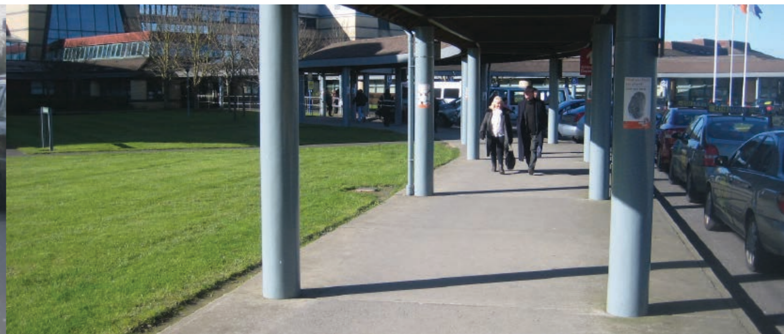
05 Covered pedestrian route forming approach to main entrance of Tallaght Hospital.
