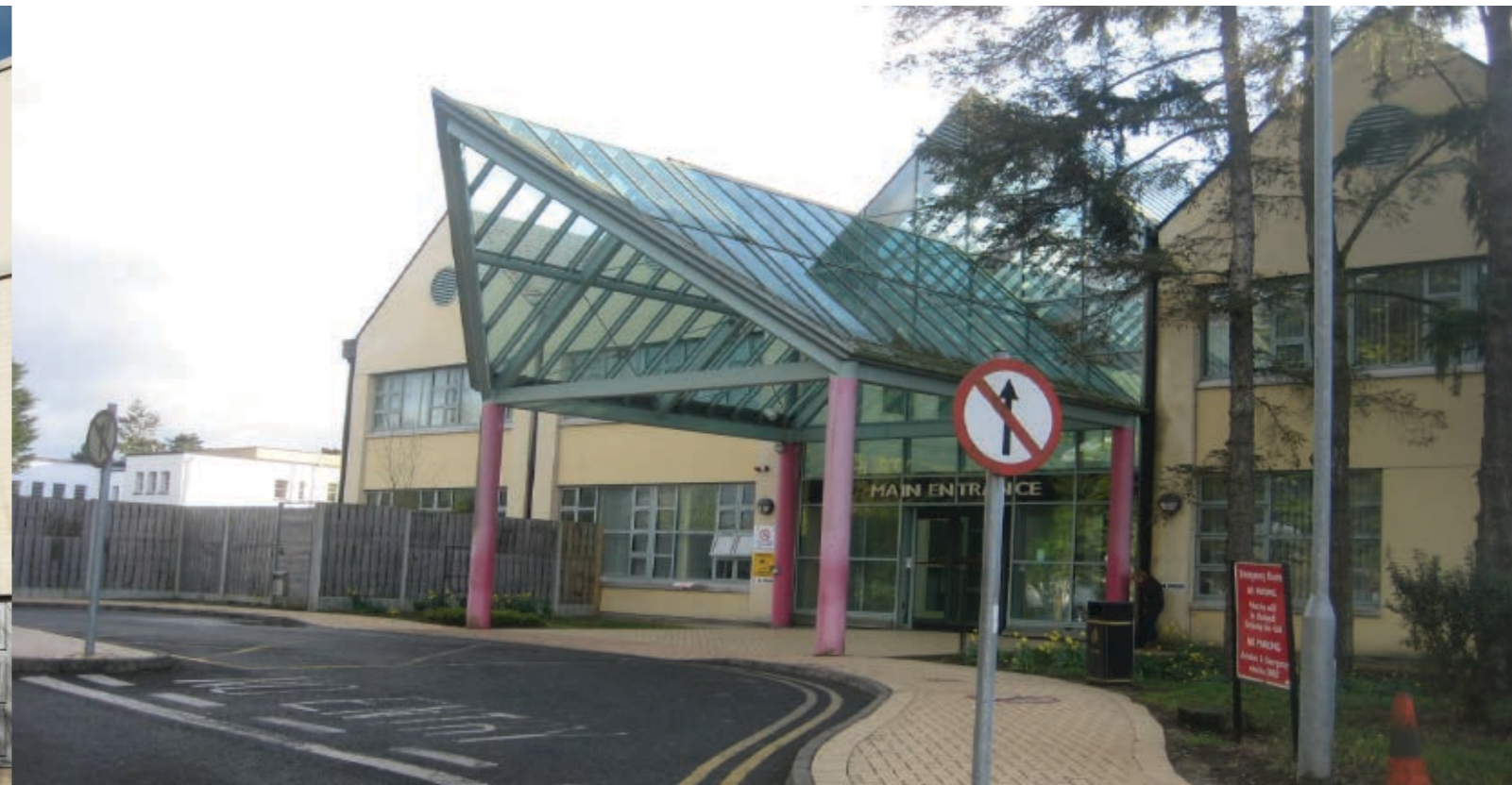
02 Main public entrance to Naas Hospital, Naas, Co. Kildare.
