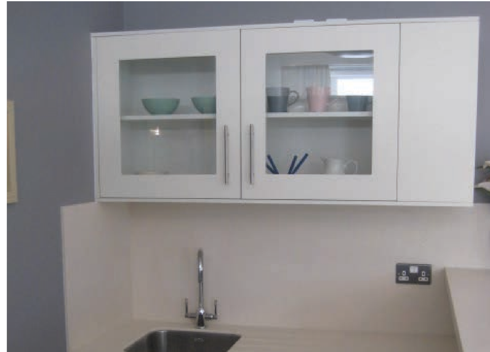
11 Kitchen units in day room, inpatient ward, Connolly Hospital, Dublin.
