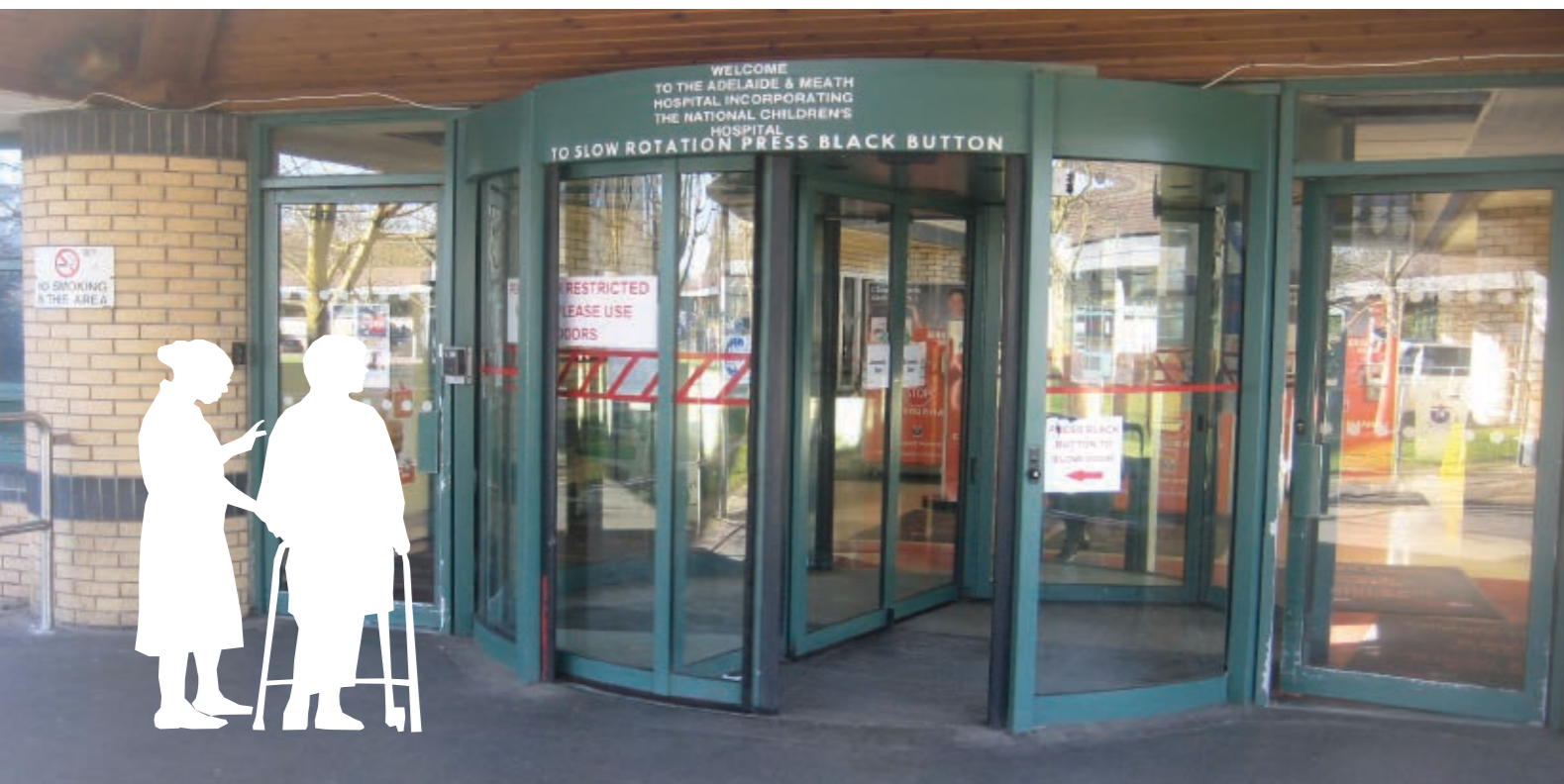
04 Main entrance door to Tallaght Hospital, Dublin, Ireland.
