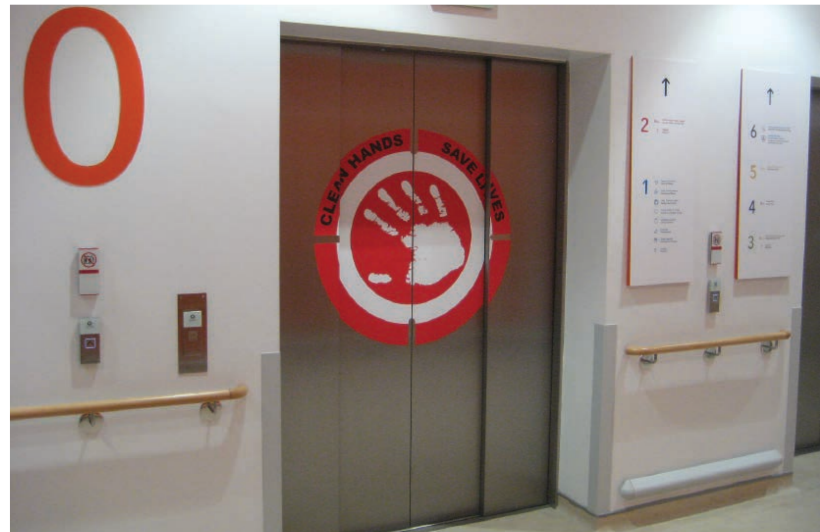
13 Passenger lift, MISA Building, St. James's Hospital, Dublin, Ireland.
