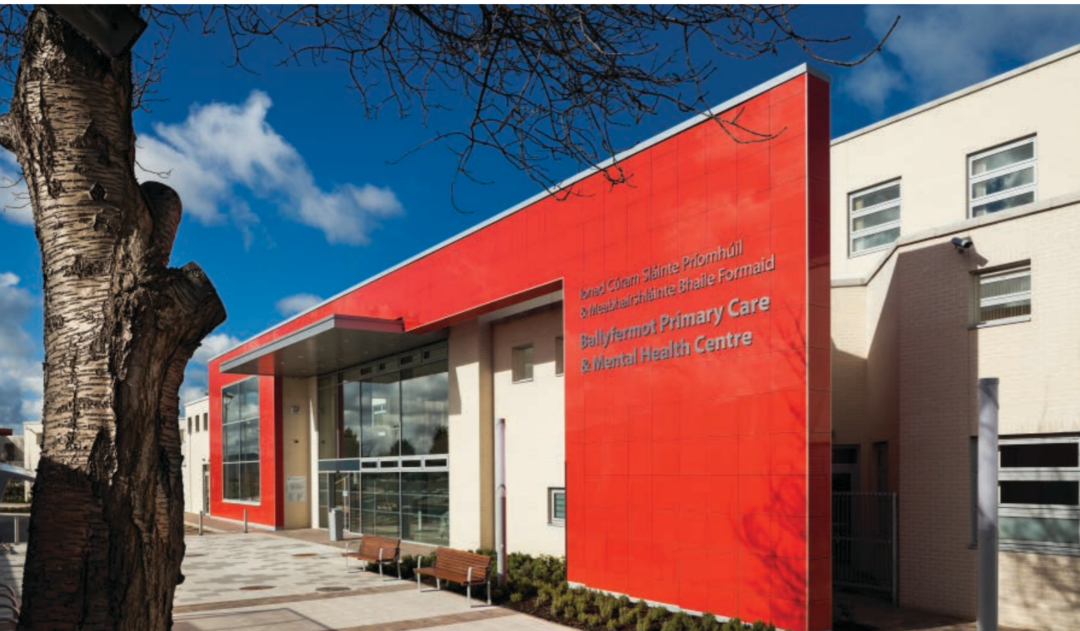
01 Ballyfermot Primary Care and Mental Health Centre, Ballyfermot, Dublin 10, Ireland.
