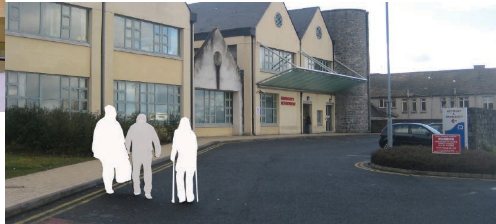
12 ED approach and entrance, Naas Hospital, Naas, Co. Kildare, Ireland.
