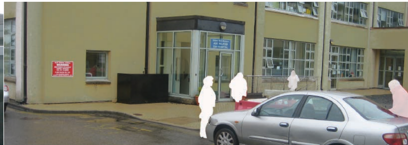
17 Day Service approach and entrance, Naas Hospital, Naas, Co. Kildare, Ireland.
