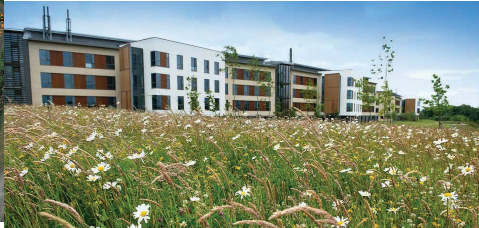
02 View to natural landscaping surrounding South West Acute Hospital, Enniskillen, Co. Fermanagh, Northern Ireland.
